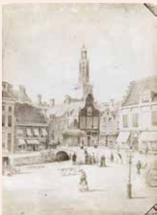
View of the Sint Jacobstraat and the Naauw (probably from the artist's living room), circa 1860.
