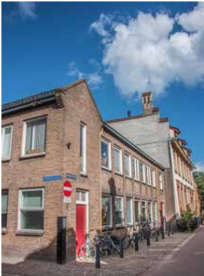
The current situation on the corner of the Bollemansteeg and the Bagijnestraat, where the Stedelijk Gymnasium was formerly located.
