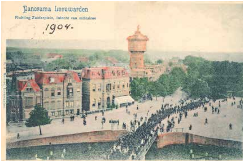
View of the Zuiderplein, with the military parade. On 22 December 1888 a modern water supply system could finally be officially put into service. The construction of the water tower on the Zuiderplein, the breaking up of the streets in order to lay the pipes and the placing of a fountain on the Hofplein - all this could not have escaped Margaretha's notice. Coloured postcard, circa 1900.
