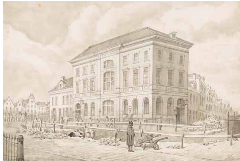
The filling of the Wortelhaven and the Eewal in 1884. An increasing stream of complaints led the municipality to fill a number of canals, many of which were of medieval origin. Margaretha witnessed the filling of the Eewal in 1884. To acquire the earth to fill it, the municipality had part of the northwestern bulwark dug up.
