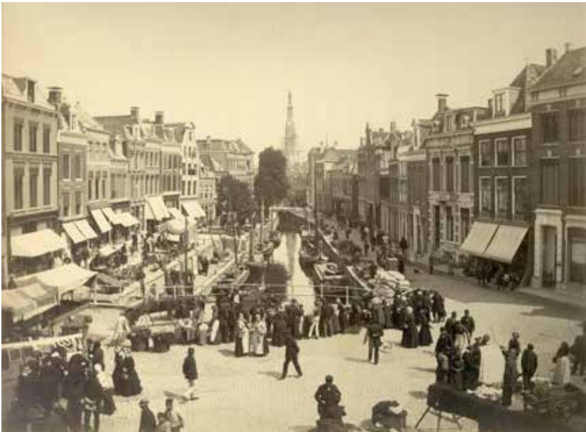
The Kelders and surroundings in 1884, as seen from De Brol, with in the background the Bonifatius tower, still behind scaffolds. Margaretha, who lived close by, undoubtedly stood and watched the construction of the Bonifatius Church between 1882 and 1884.
